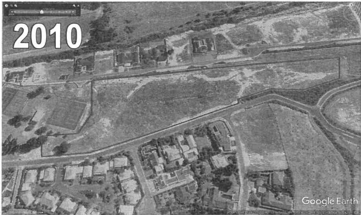
Figure 9: Erf 1692 during 2010, showing ongoing vegetation recovery, exotic Pinus and Eucalyptus species removed
